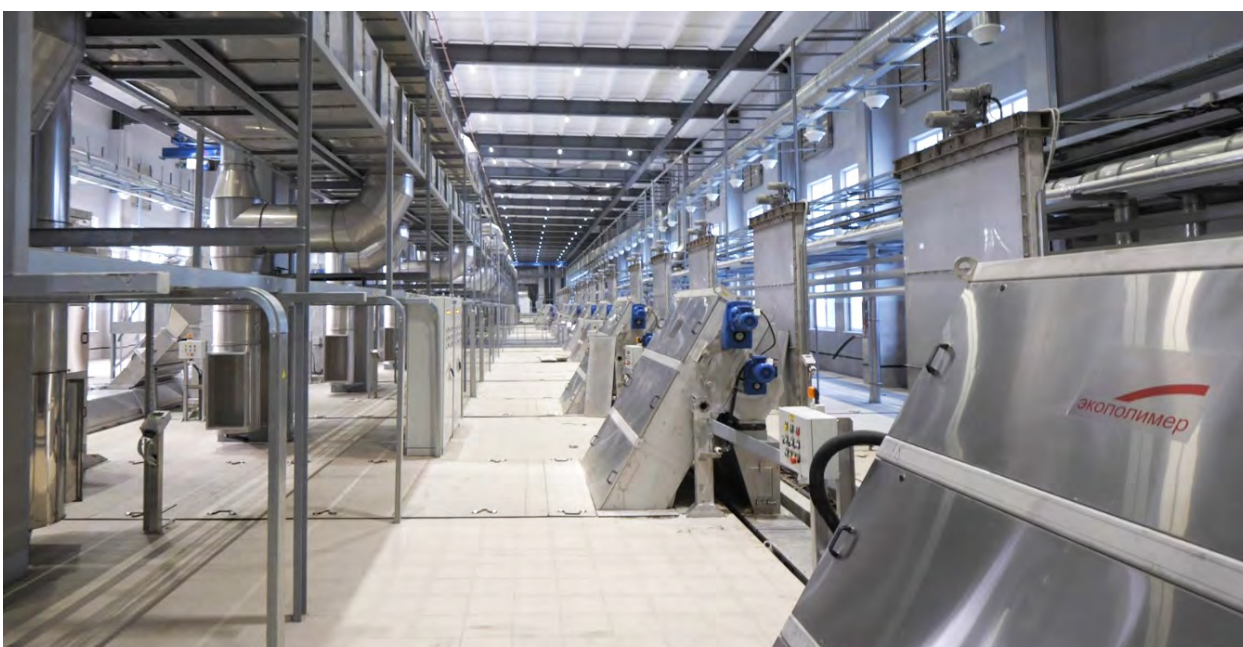
24 «MY MET» complexes at the Lyuberetsky wastewater treatment plant of JSC «Mosvodokanal». Capacity 3 000 000 m 3 /day.
